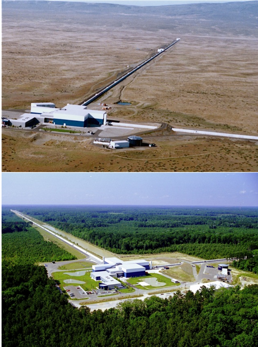
Figure 2. Aerial photograph of the LIGO observatories at Hanford, Washington (top) and Livingston, Louisiana (bottom). The lasers and optics are contained in the white and blue buildings. From the large corner building, evacuated beam tubes extend at right angles for 4 km in each direction (the full length of only one of the arms is seen in each photo); the tubes are covered by the arched, concrete enclosures seen here.
