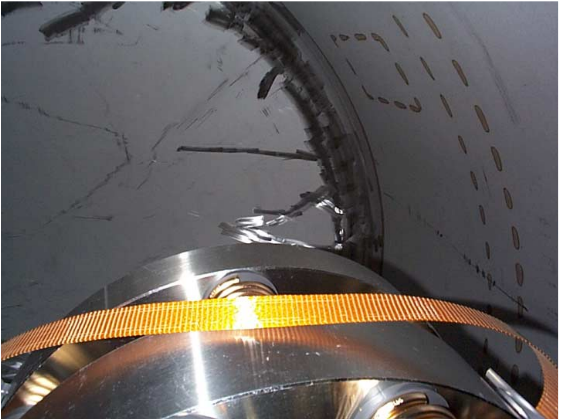
WBSC 2 Feb 4, 2000: 147. NE stack, viewed from E
