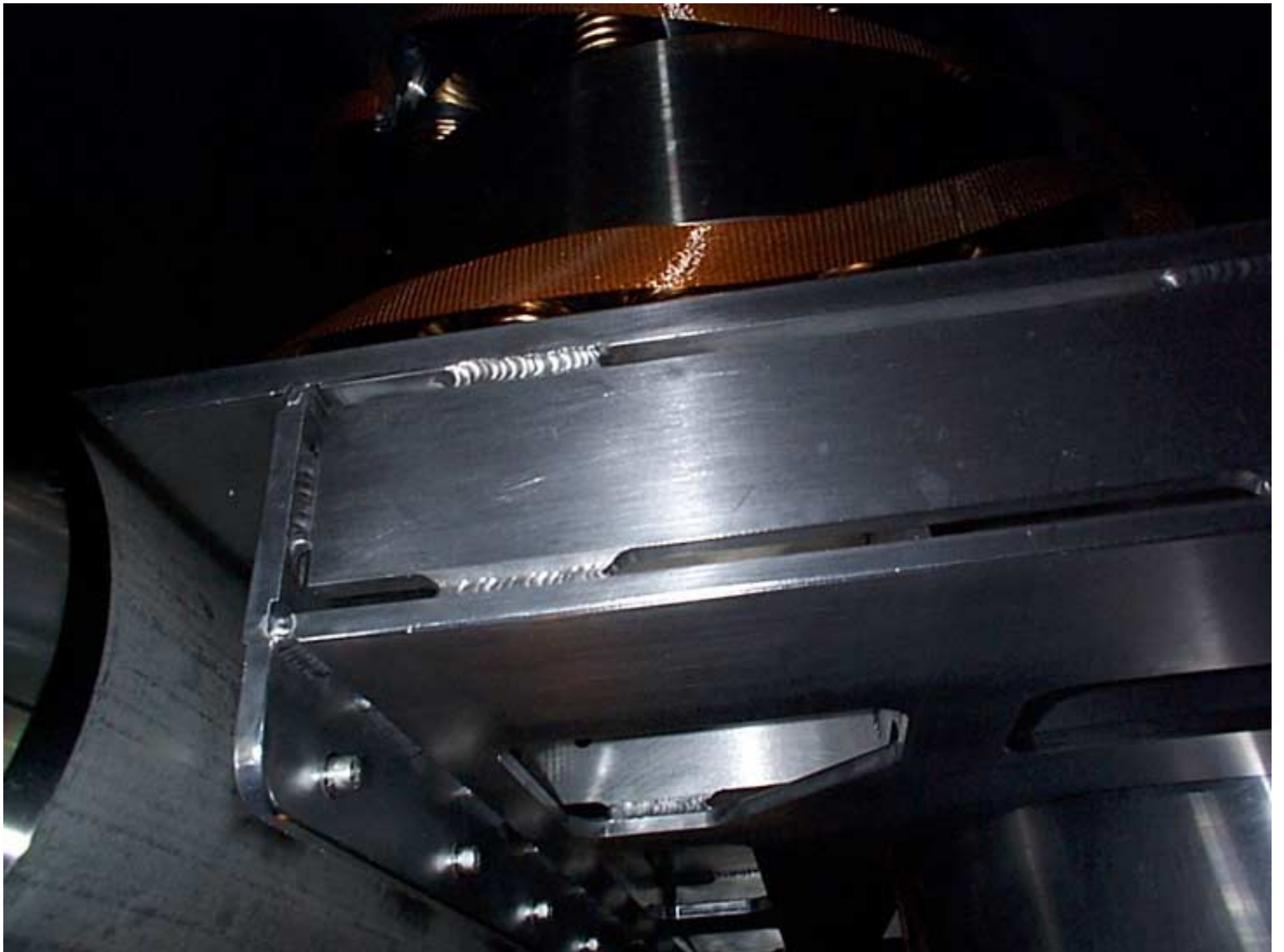
WBSC 2 Feb 9, 2000: 161. NE stack, viewed from N
