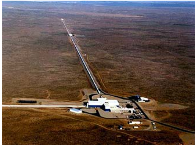
Figure 1.1: LIGO Hanford Site [2]
