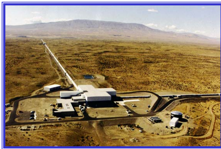
Figure 1 Overhead view of Hanford detector. Notice the L-shape and the immense 4km arms.
