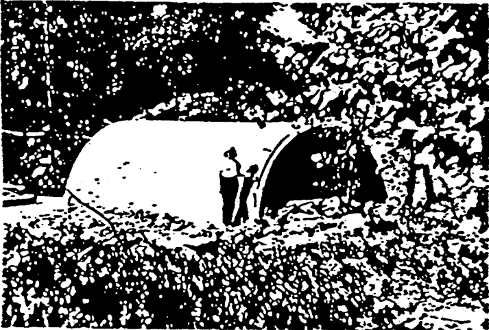
AIR-O-FORM™ SAVES CONSTRUCTION TIME. This 14 foot span by 7 foot high arch was completed in six hours, using a four man crew.
