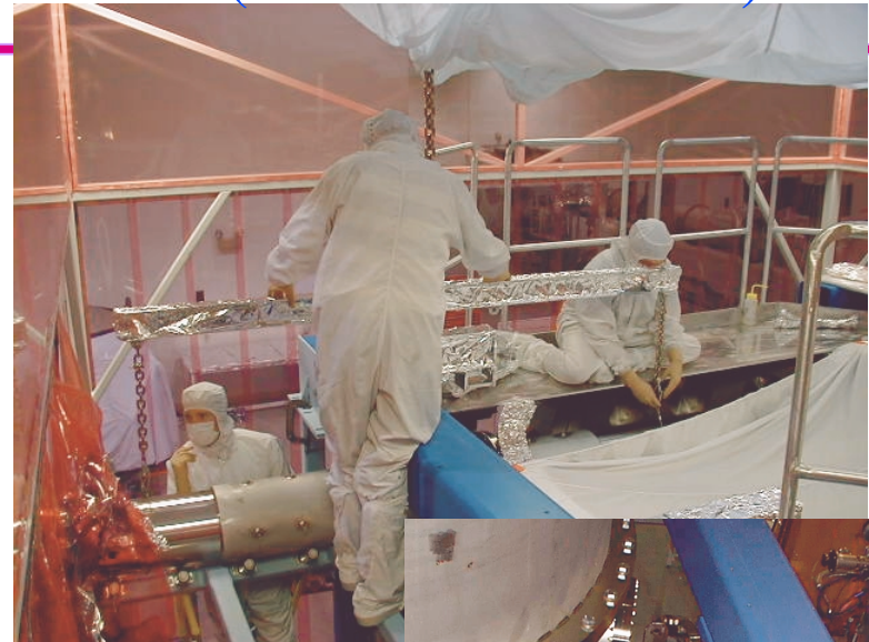
Support Tube Installation (Hanford WBSC7)
