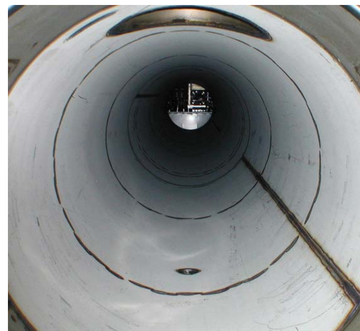
View of the interior of the current tube 16
