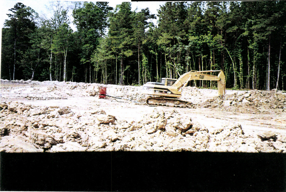
12. Southeast Arm at station 130+00 looking west at excavating fill for placement on end station.
