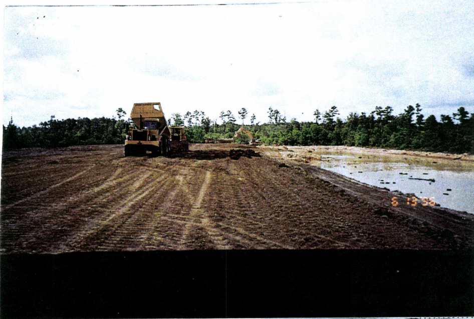
10. Southeast arm at station 128+00 looking SW at spreading and compacting fill near end station
