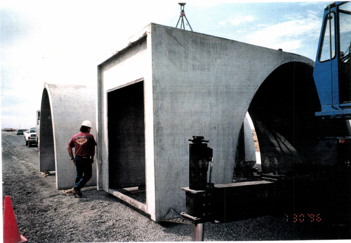
Different views of the beam tube enclosure modules as they are set on to the beam tube access road in preparation for the mock up demonstration.
