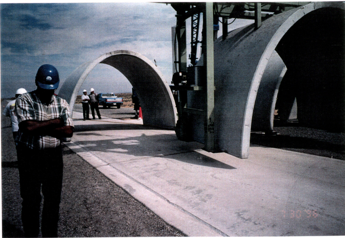
Both type "C" beam tube enclosure modules are set on to the beam tube support slab for the mock up demonstration.
