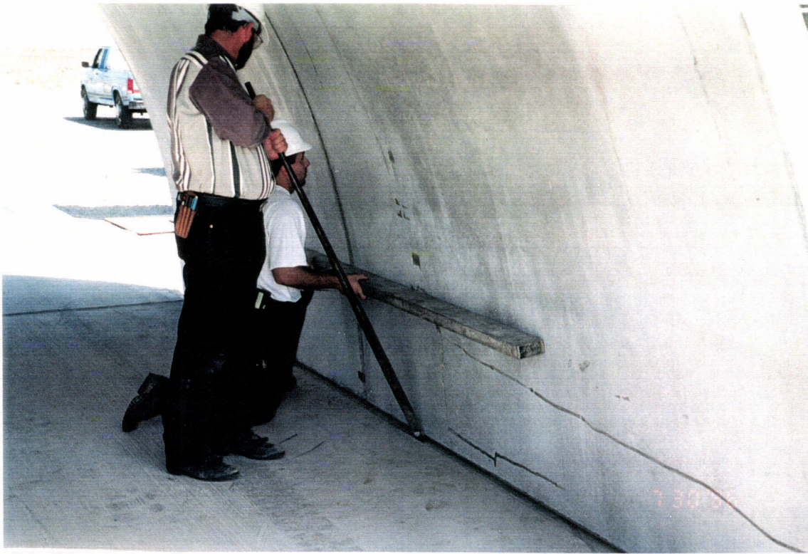
Alignment of the beam tube enclosure modules is verified as acceptable.
