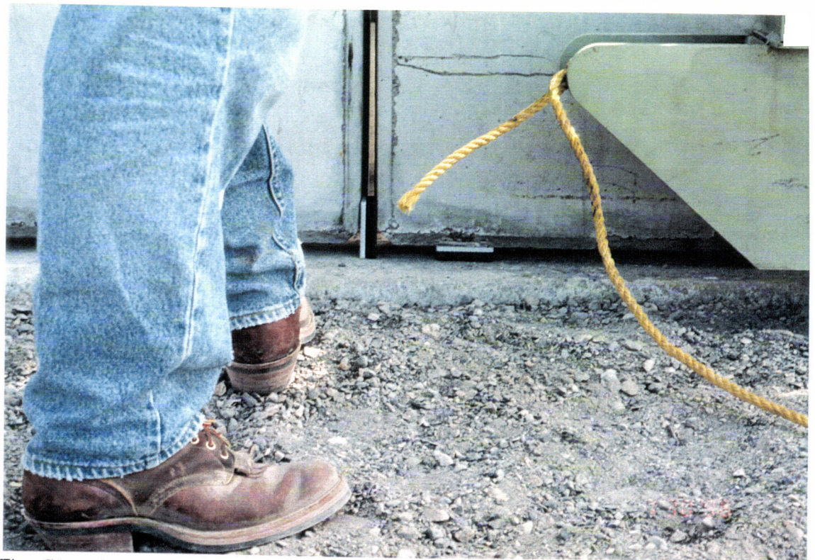
The fit up between beam tube enclosure modules is verified as acceptable. The shim between the enclosure modules is serving as the required spacer.
