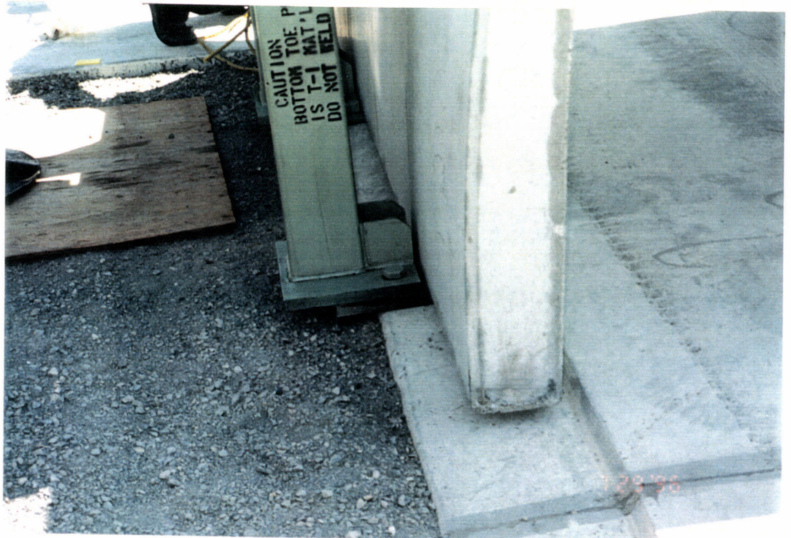
View of the beam tube lifting device to show the beam tube enclosure setting on to the beam tube support slab alignment groove.
