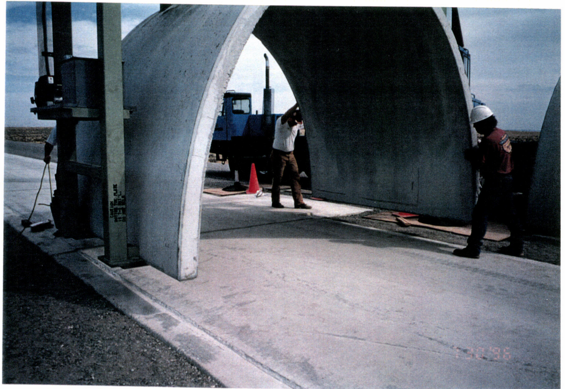
Beam tube enclosure module is set on to the beam tube support slab for the mock up demonstration.
