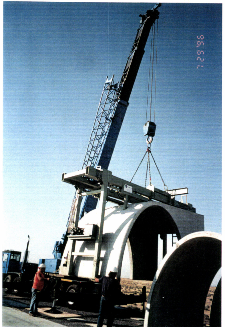
Beam tube enclosure module is set on to the beam tube support slab for the mock up demonstration.
