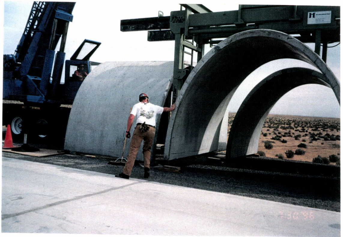
Set up of the beam tube enclosure lifting device for lifting the enclosure module
