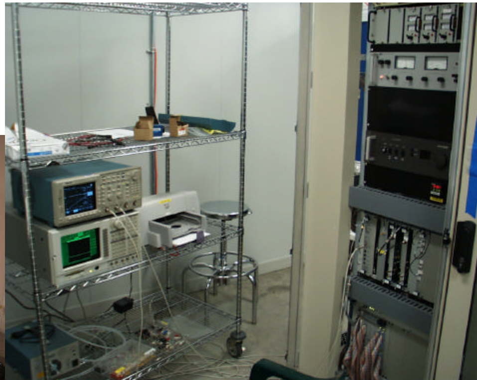
PSL control electronics
