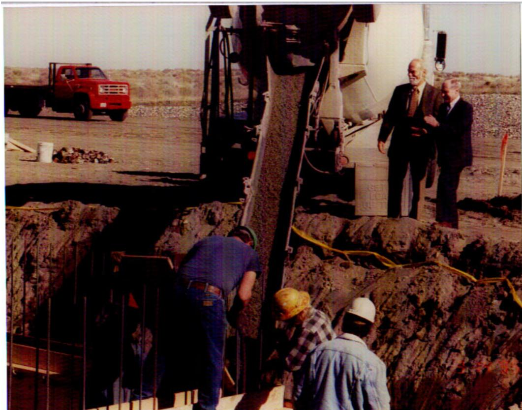
**FIGURE 1. The first concrete is poured at LIGO. Dr. Barry Barish (Caltech) and Dr. Dave Berley (NSF) watch as concrete is poured for the Termination Valve Anchor Foundation on the southwest arm Mid-station at Hanford. (March 1996)**
