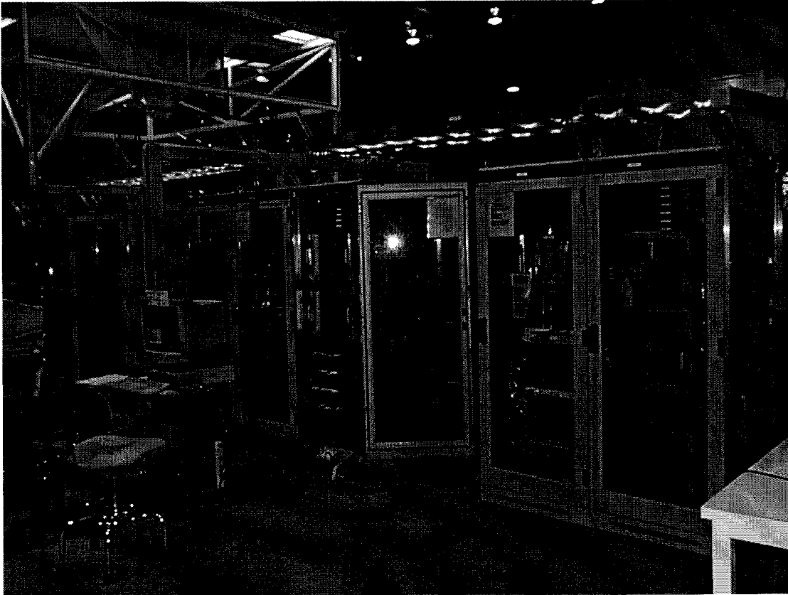
FIGURE 4. Mode Cleaner Electronics Racks (Hanford two kilometer interferometer).
