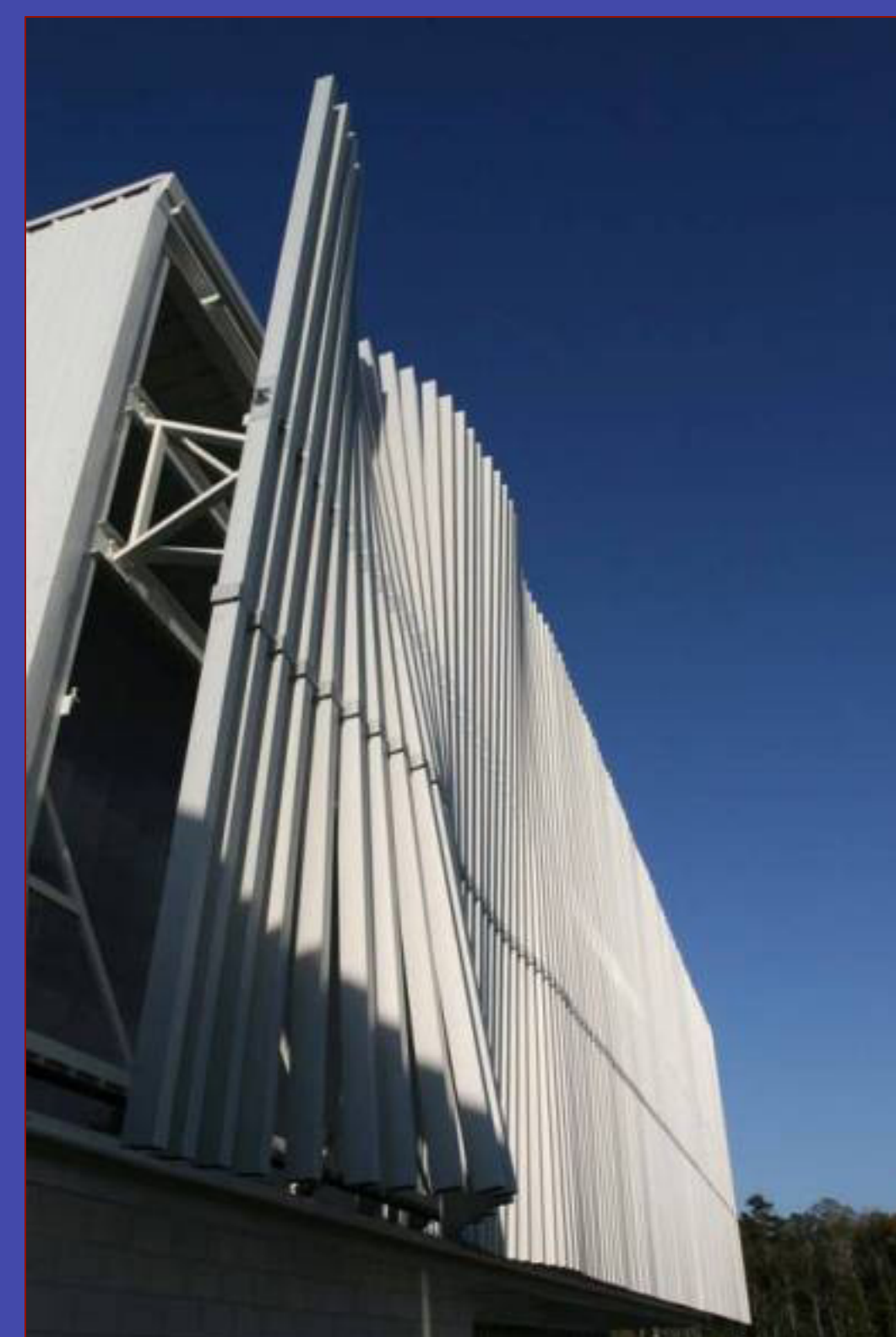
Left: The Wave Wall attached to the front of the SEC produces moving waves in the wind.
