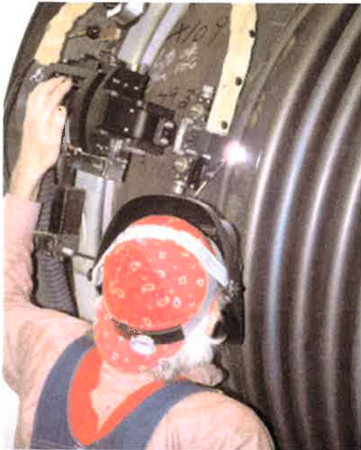
Figure 9 - Circumferential Seam Welding
