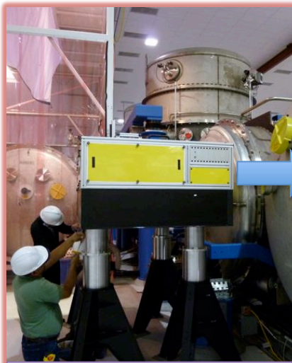
Squeezer table craned to its final location
