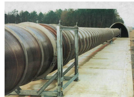
LLO Beamtube: Side view of exposed beamtube during construction at LLO.
