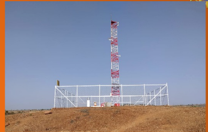
Weather station at the LAO site
