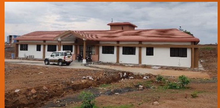
Site office at the LAO site
